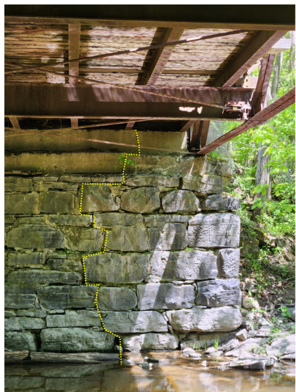
Photo 10: Crack in bearing seat, ballast wall and masonry indicative of differential settlement (East Abutment).
