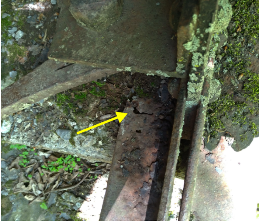
Photo 20: Severe corrosion and perforation in bot. chord (south chord, east end, looking down)
