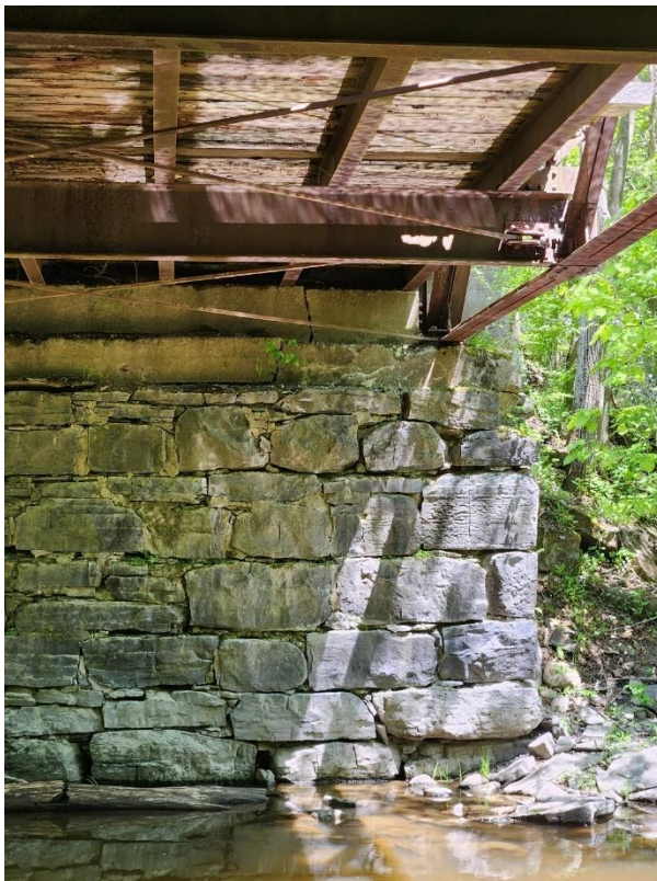
Photo 10: Crack in bearing seat, ballast wall and masonry indicative of differential settlement (East Abutment).
