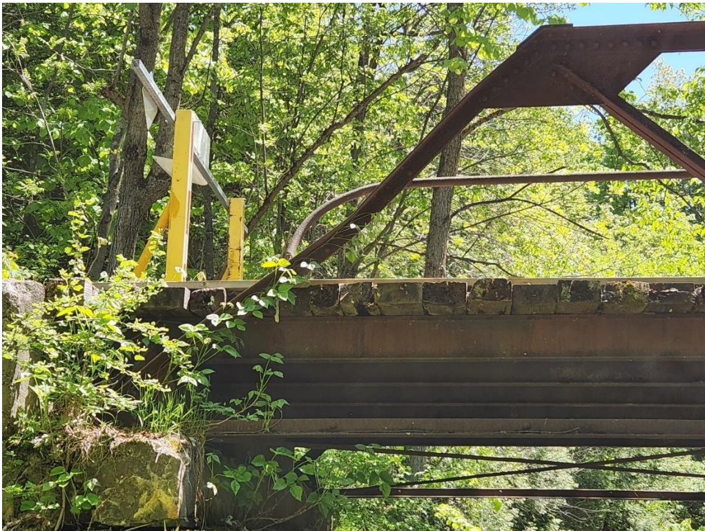
Photo 18: North compression chord buckling at east downturn
