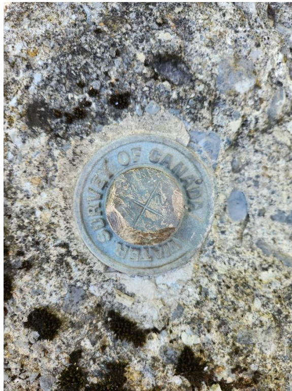
Photo 12: Existing benchmark on east ballast wall.
