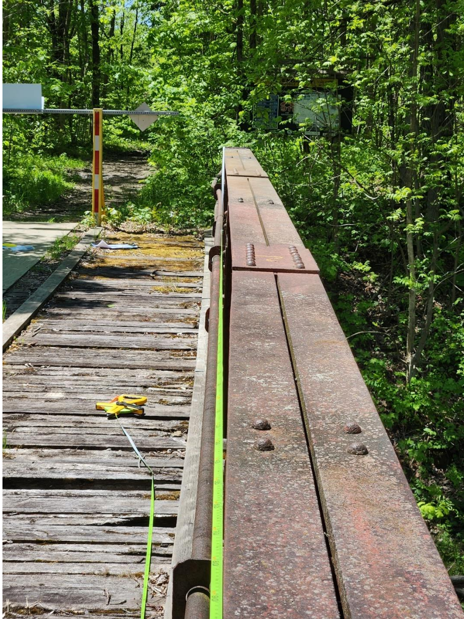
Photo 19: Global buckling of north truss panel.
