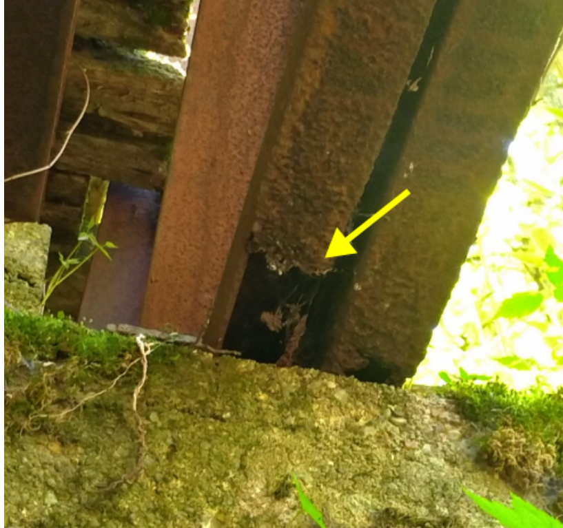
Photo 21: Severe corrosion and perforation in bot. chord (south chord, east end, looking up)
