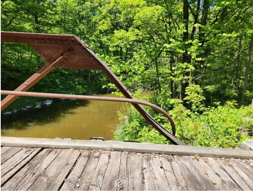
Photo 17: North compression chord buckling at east downturn and damaged railing.
