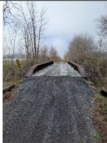
Bridge crossing with new aggregate surfacing. Potential liability due to no guardrail and minimal mats to assist users to cross floor grating.
