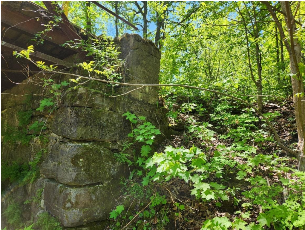
Photo 16: Northwest embankment and eastern bearing seat and ballast wall.
