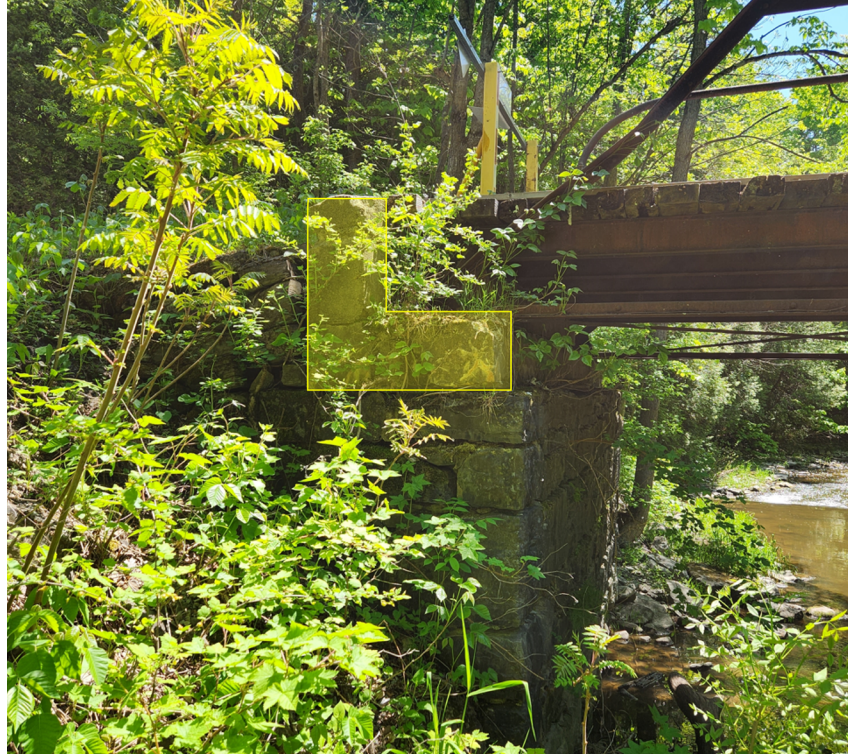
Photo 9: Outline of concrete bearing seat and ballast wall (East Abutment).
