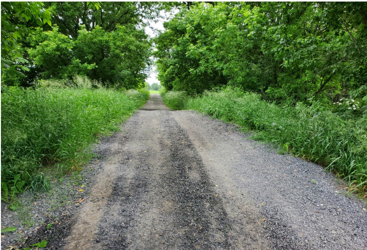
Photo 4 Wearing surface: loss of granular material throughout
