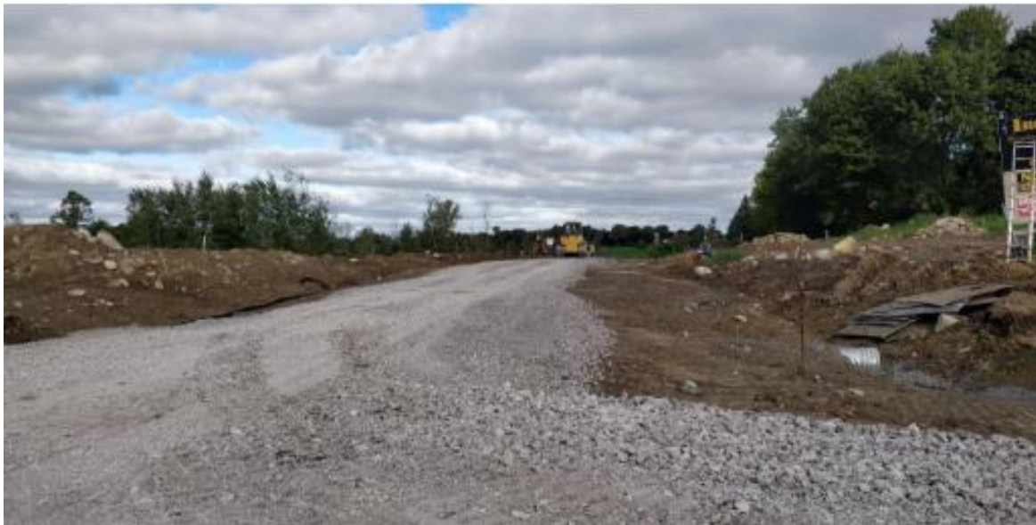
200mm (thickness) lift of Granular 'B' on South Portion of Sapphire Drive (approx. 66m in length; Looking North), September 23, 2022
