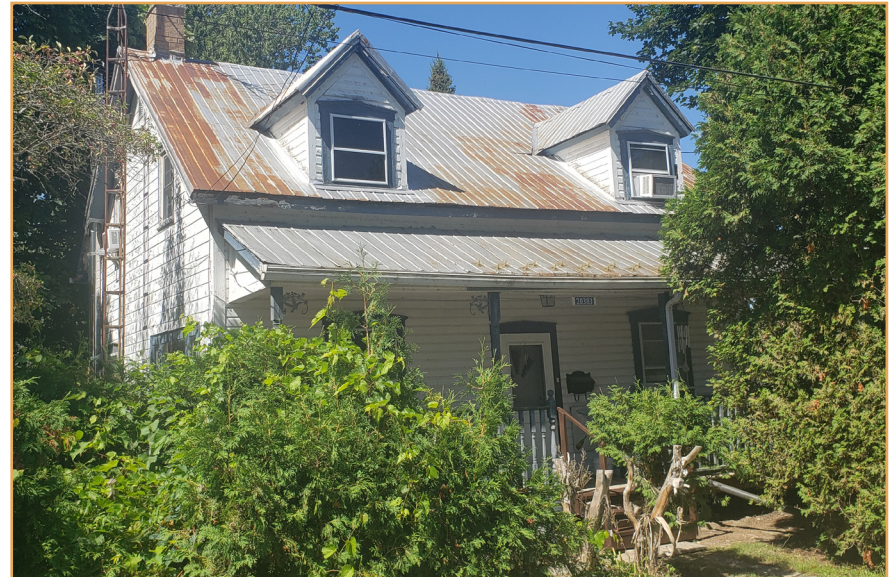
/ BUILDING D 20383 Old Montreal Road
