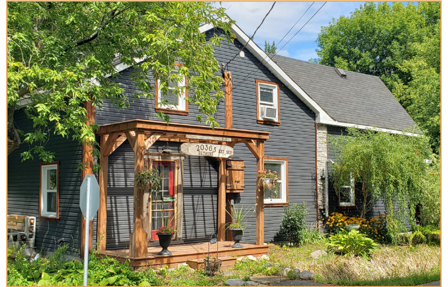
/ BUILDING F 20365 Bethune Street
