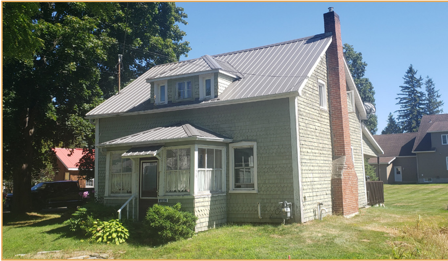
/ BUILDING C 20382 Old Montreal Road
