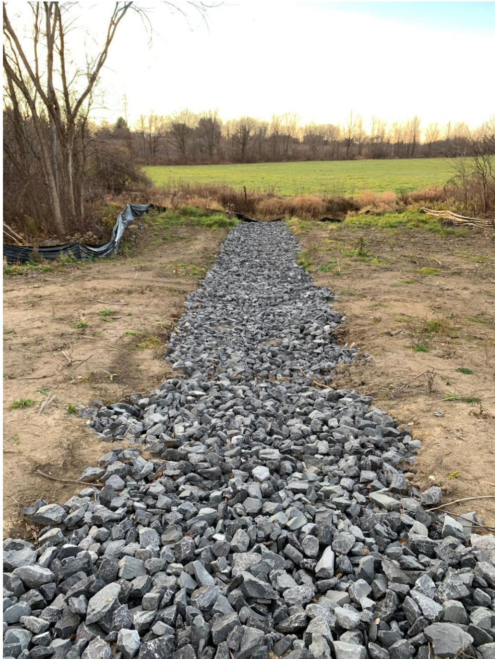
Photograph 17: SWM Facility Overflow Channel
