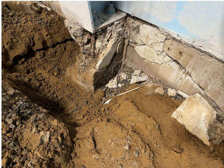
Photo 1: Pier damage
